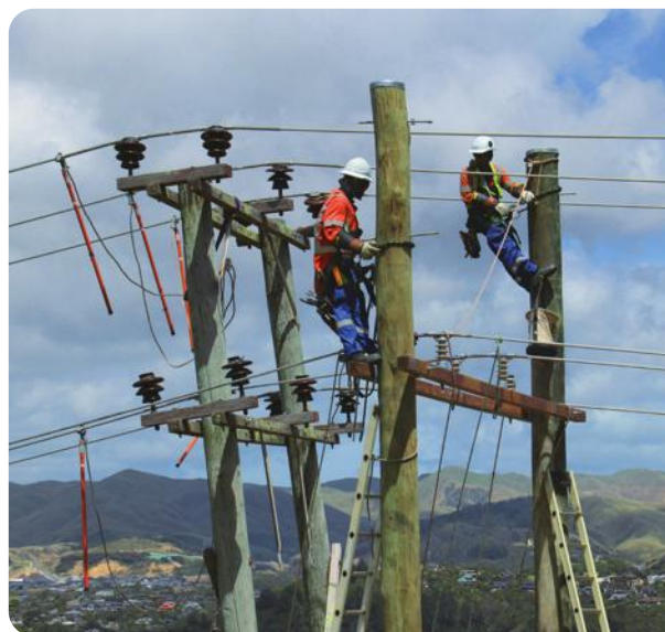
▶ WELL workers repair high-voltage poles to upkeep network reliability.
