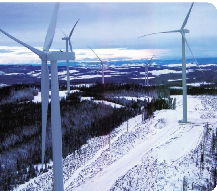
Canadian Power's Okanagan wind farm supplies renewable electricity to British Columbia.
